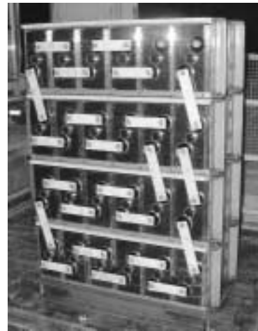
写真5 FMU-S-1000-12-24S耐震試験体外観 Photo.5 Overview of FMU-S-1000-12-24S battery group
